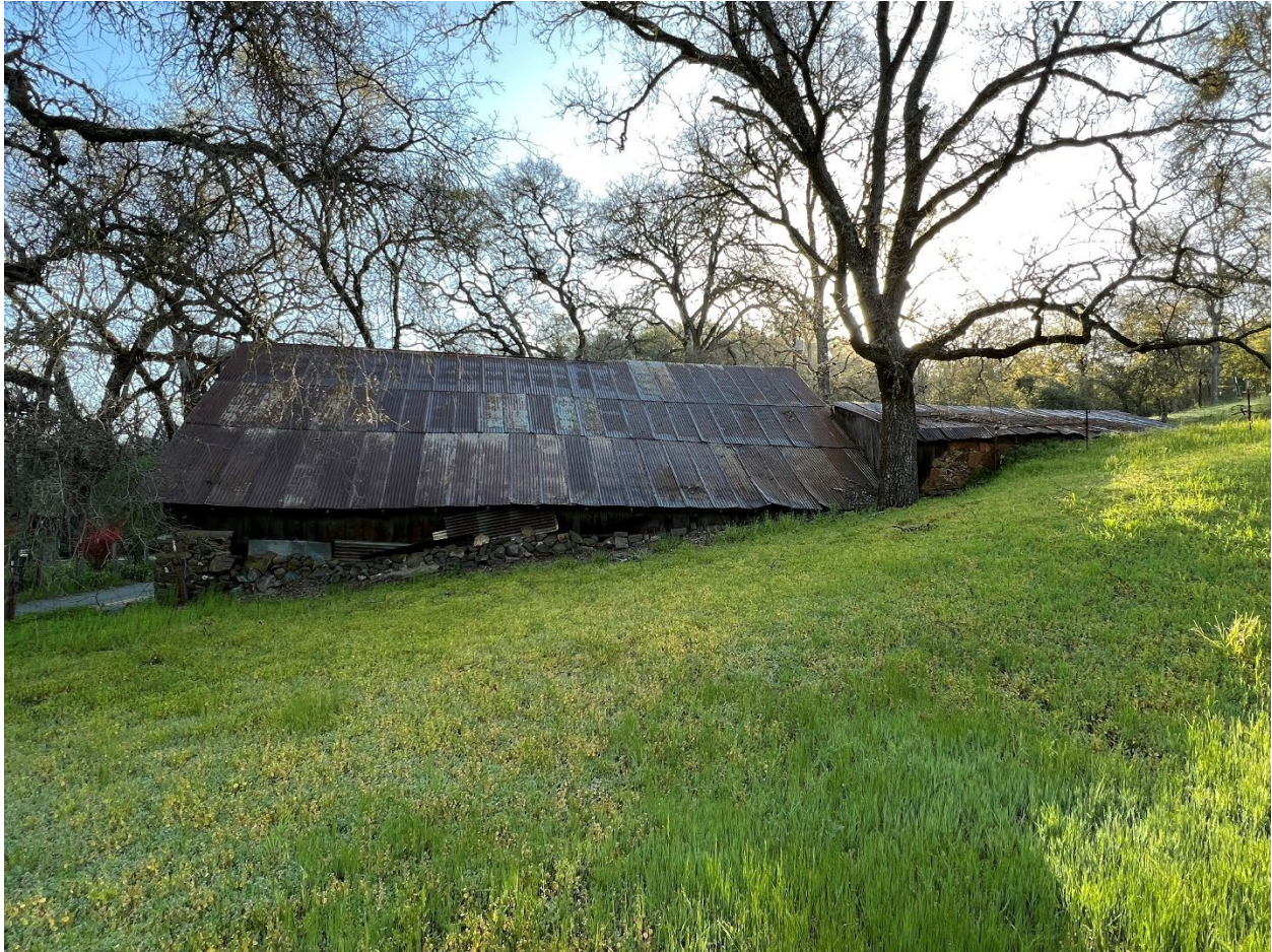
Photo #1: View of the western façade of the Winery building showing it cut onto the slope of the ground.
