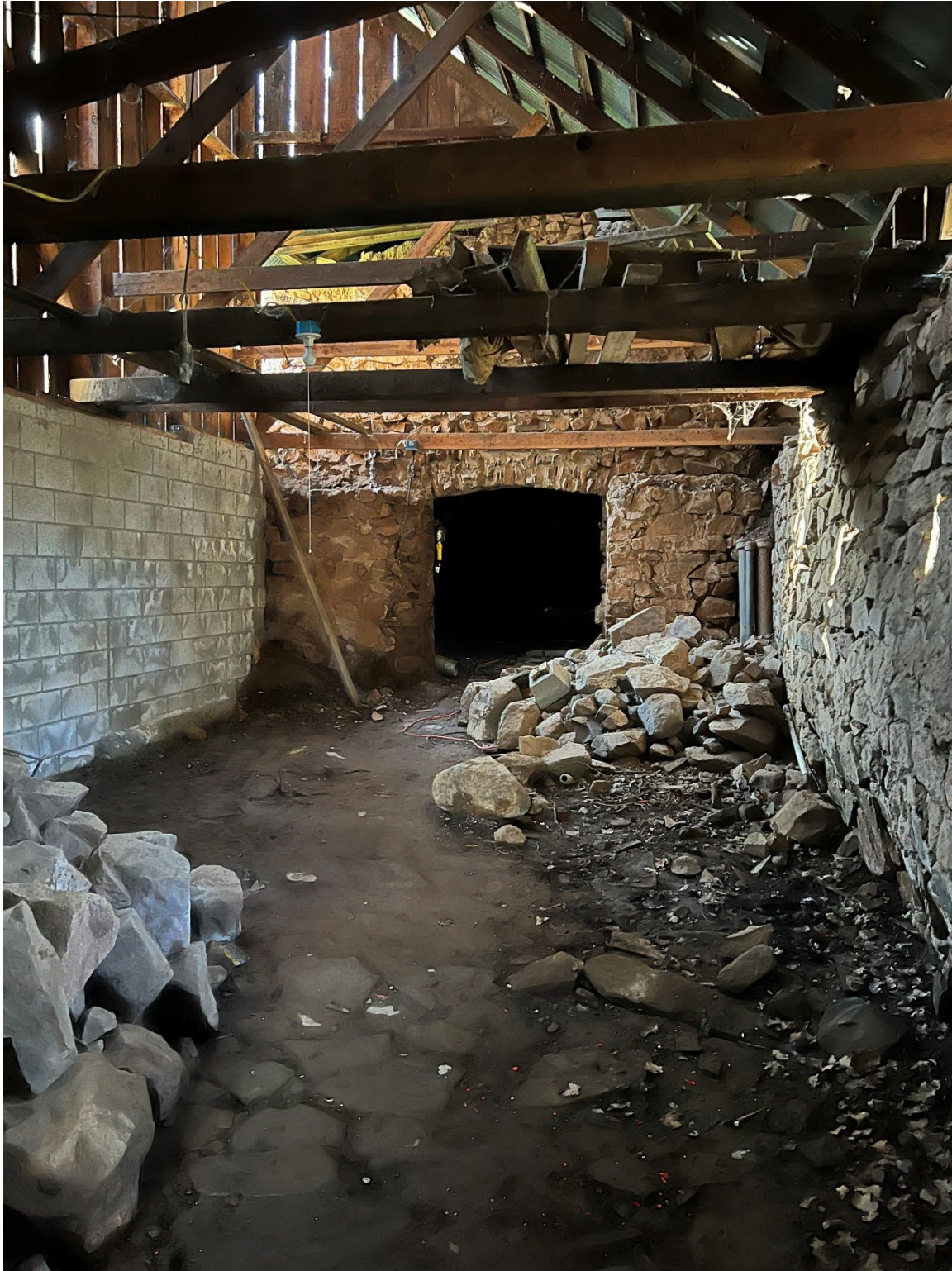
Photo #16: Interior view of the front portion of the Winery building.
