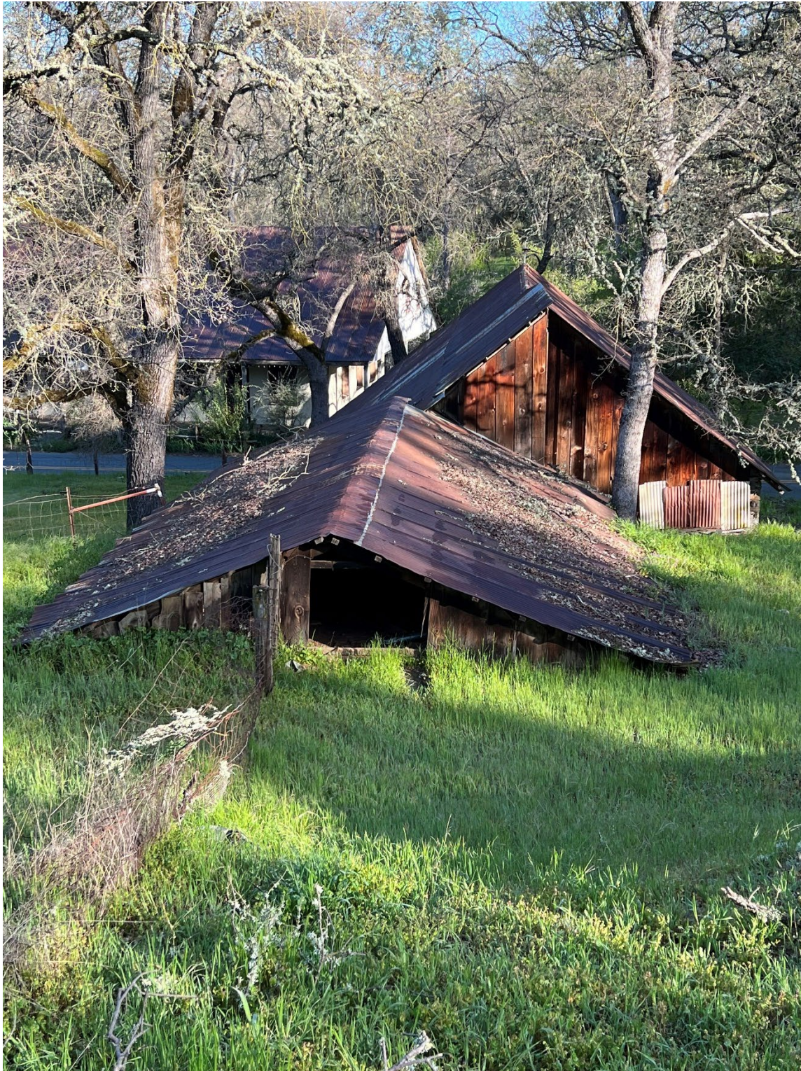
Photo #14: View of the rear façade of the Winery building.
