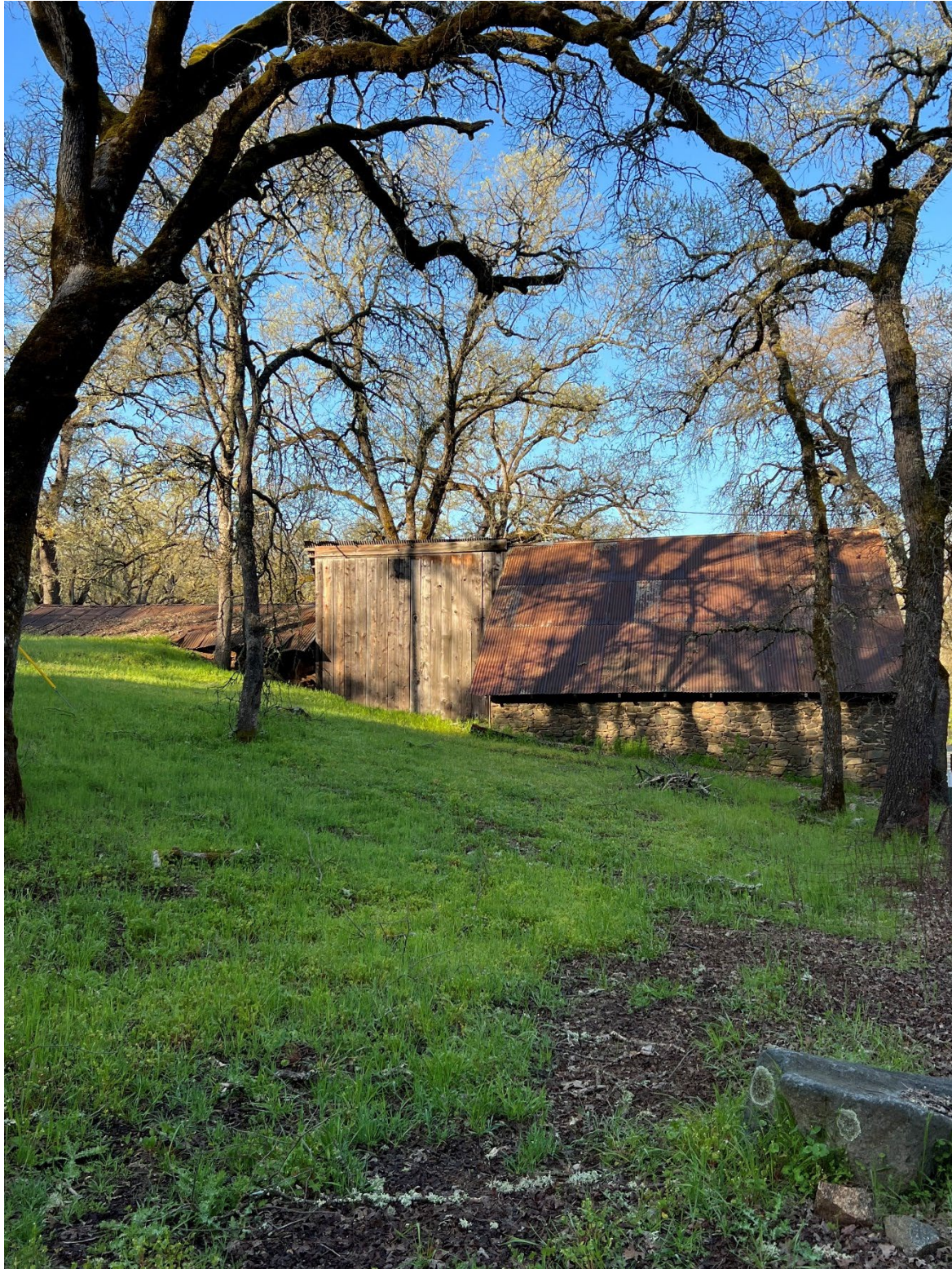
Photo #15: View of the eastern façade of the Winery building.
